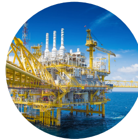
Pilot injection application
